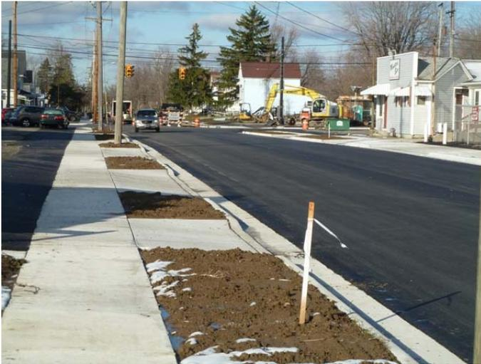
This project reconstructed (full depth) 2100 feet of street with curbs, drive approaches, ADA wheel chair ramps, and drainage on South Metcalf between the railroad underpass and Kibby Street. The cost of the project was \$637,716.51 and was paid for with \$573,944.86 from OPWC State Issue I funds and \$63,771.65 from CDBG Funds (90/10). The project was a continuation of improving the main corridors into the city.
