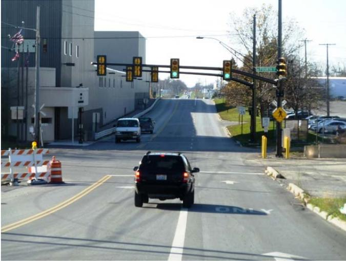
This project was originally scheduled to be completed in 2010, however a longer than expected lead-time on the traffic signal equipment pushed the project into 2011. The intersection was upgraded with mast arm poles, pedestrian facilities, drainage, and pavement resurfacing. The improvements aid the high number of pedestrians that cross S. Metcalf St. on the south leg of the intersection with overhead lighting; visible
