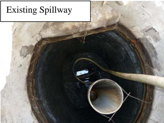
2008, Ohio Department of Natural Resources (ODNR) conducted a safety inspection of Schoonover Dam. Following the inspection of our class III dam, ODNR required several remedial measures be taken by the City to ensure the dam remains safe. The remedial measures included providing an emergency spillway, investigate signs of seepage, repair and rebuild eroded downstream slope, and repair of erosion on the upstream slope. Following a Field Reconnaissance and
