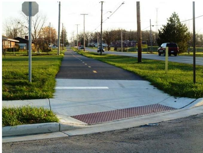
side. The total length of the 10-foot wide asphalt path is 0.75 miles. The cost of the project was \$229,185.29 and was funded through ODOT CMAQ and CDBG funds at an 80/20 split. Like the Cable Road Sidewalk Project, the City was reimbursed \$2,802.63 for construction inspection costs (labor).
