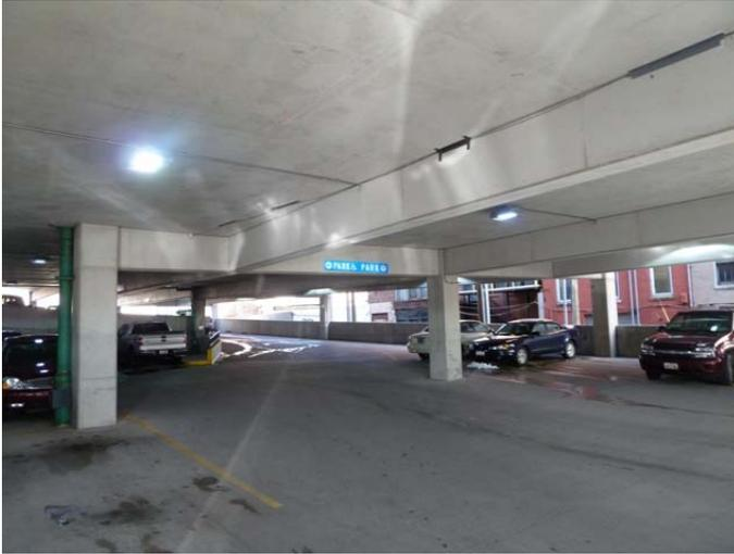
This project also continues the energy savings pursuits of the City by replacing all T12 fluorescent tube fixtures with T8 and just over 150 HID Garage Luminaries with LED Garage Luminaries. The light quality was also improved in the parking garage making it a brighter, safer, and more inviting place to park your vehicle. The total cost of the project was \$123,570.66 and made possible through an RZ Bond, which is a low interest rate loan through the EECBG program.
