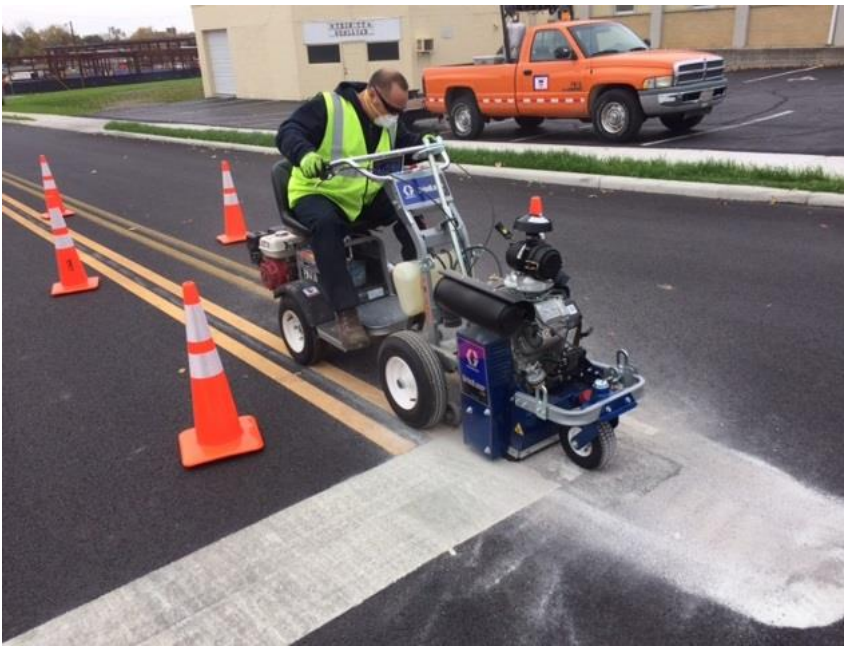
Darren Barnett using the hand propelled grinder to remove traffic control
